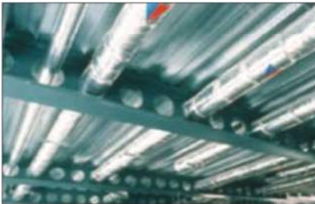
Complex Services Integration in Cellular, Long-Span Beams
