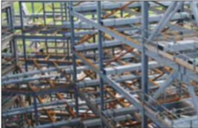
Braced Frame Construction
