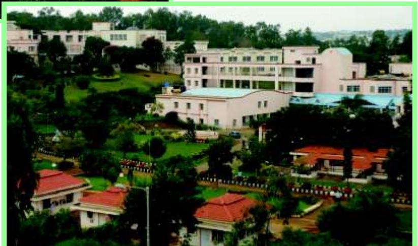
Expansion of National Institute of Unani Medicine including Ward, OPD, Pharmacy, Regimetal Therapy Block and Auditorium
