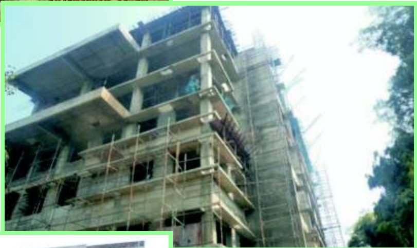
Construction of OPD Block, Lady Hardinge Medical College, New Delhi
