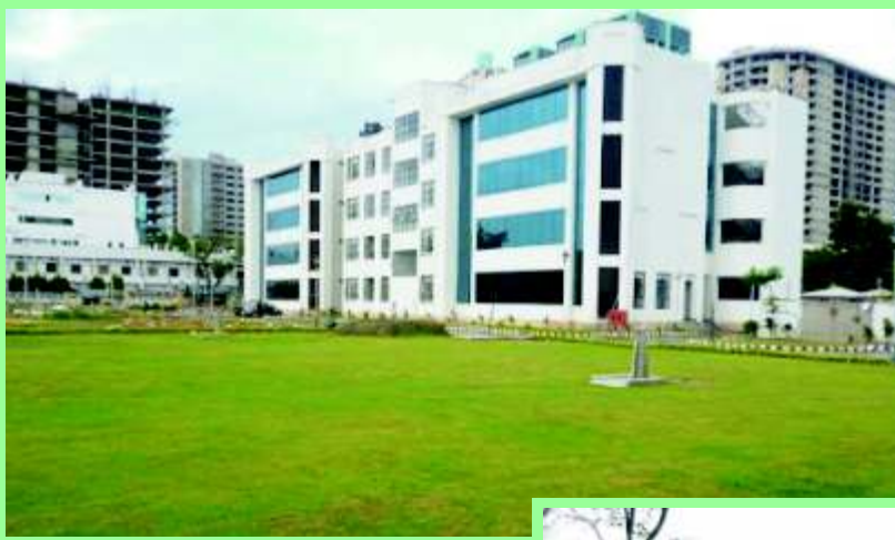
New Campus consisting of 13 Research Laboratories, Administration Block, Director's Office, Seminar Hall, Library etc. for Indian Institute of Chemical Biology (I I C B), Kolkata
