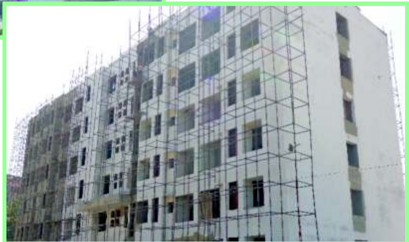
Construction of Hostel Block, AIIMS, New Delhi
