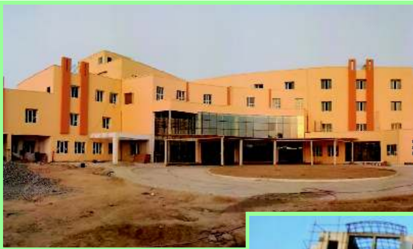
Construction of 100 bed Advanced Cancer Diagnostic Treatment & Research Centre, Bhatinda
