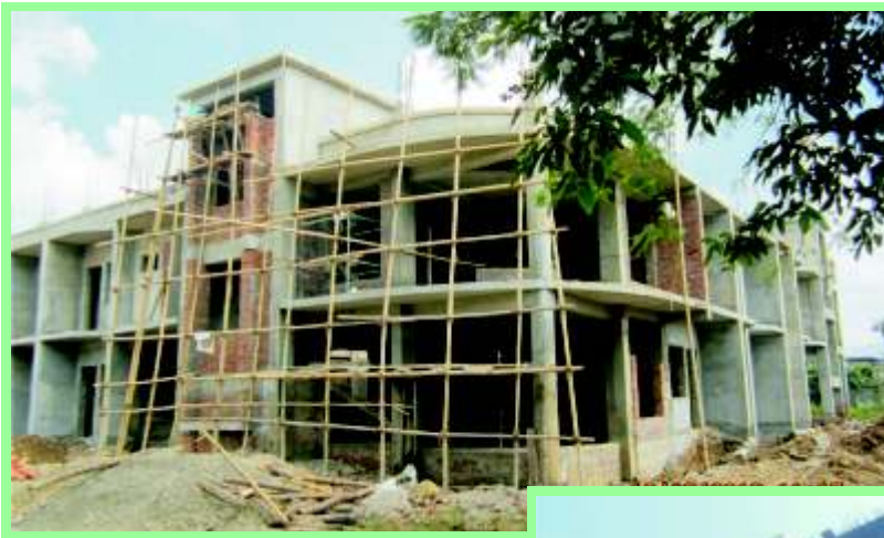
Construction of Hostels for Regional Institute of Medical Sciences (RIMS), Imphal
