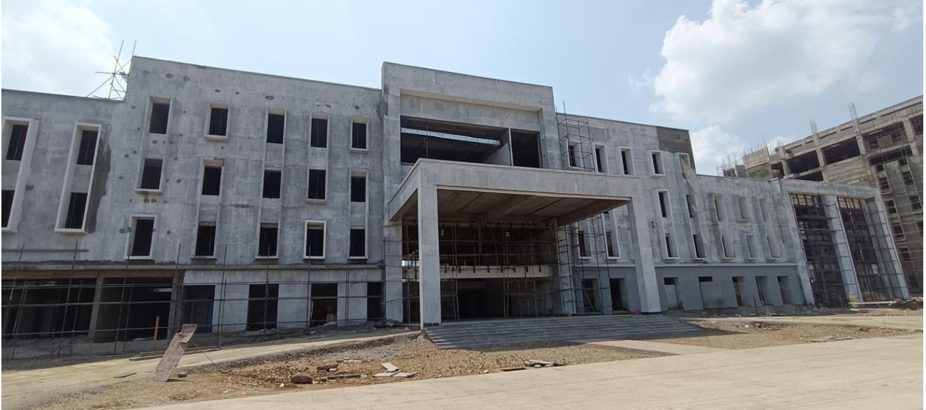
Construction of Govt Medical College at Jalgaon
