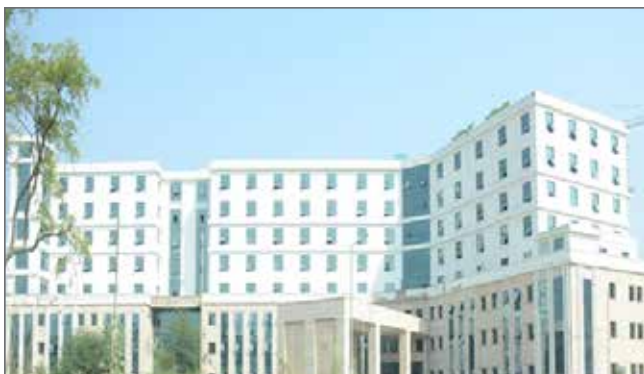
AIIMS Raebareli - Hospital Block
