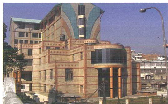
A view of 200 beded Emergency & Trauma Centre for Bir Hospital, Kathmandu, Nepal
